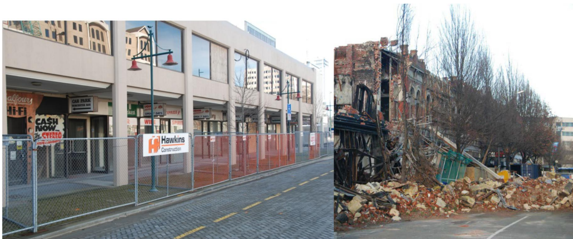
Figure 1 (Left) Businesses unable to access their premises in Christchurch CBD; (Right) Damage to unreinforced masonry facade in an historic street in Christchurch: the street remains inaccessible four years after the earthquakes. (Photo Credit: Dr Graham Tobin).
